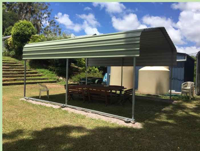
Newly erected barn at Soil & Soul, Palmwoods Community Garden
